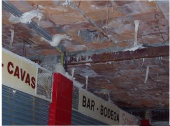
The poor state of the slab that supported the square of the urbanization El Recreo, located in the municipality of Móstoles, as well as the need to enable emergency vehicles, in particular fire trucks, to access to this area, led the city council to consider the solution of the problem by reinforcing this slab.
