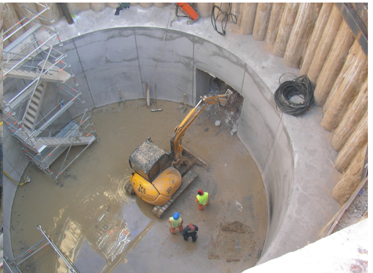
Inlet of the sewer pipe
