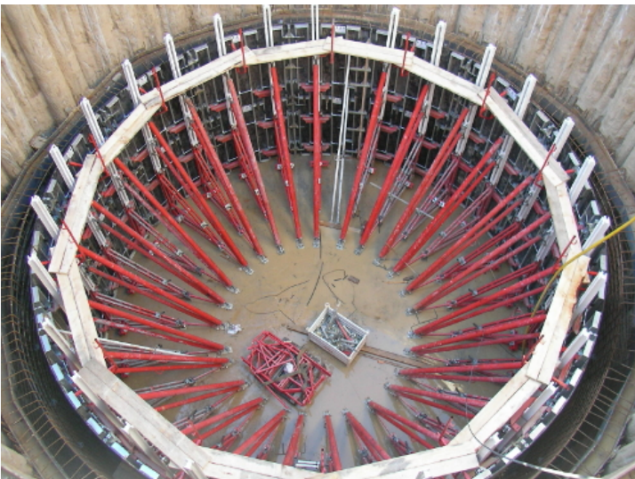
Formwork for concrete wall 4.5 m high, 1.1 m thickness
