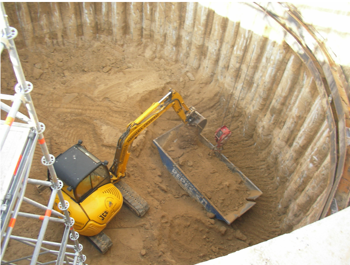
Excavation of the shaft
