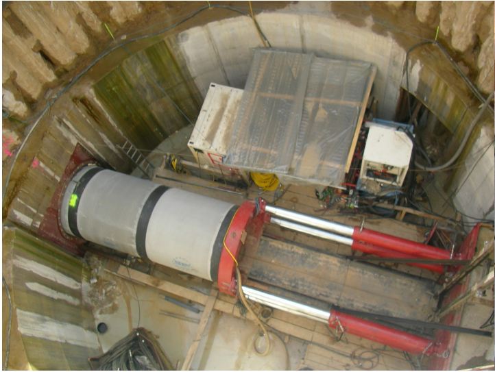
Pipe jacking, withstanding a maximum thrust of 12.000 kN
